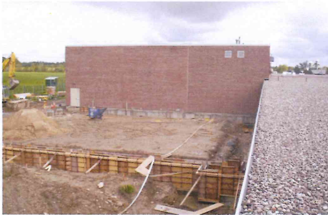
New MHS Gymnasium Foundation
