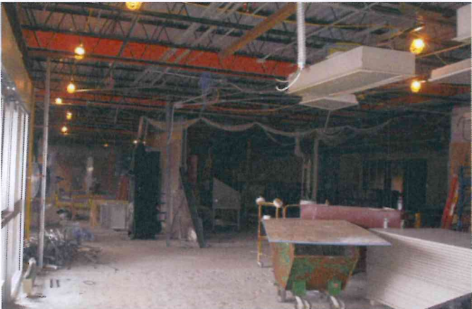
MHS Main Office Renovations Underway
