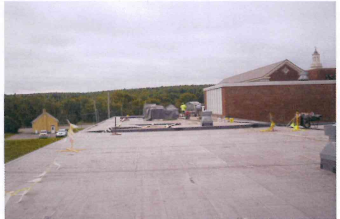
New Roof ES Wing
