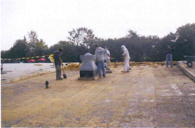
Roof Removal at ES Wing
