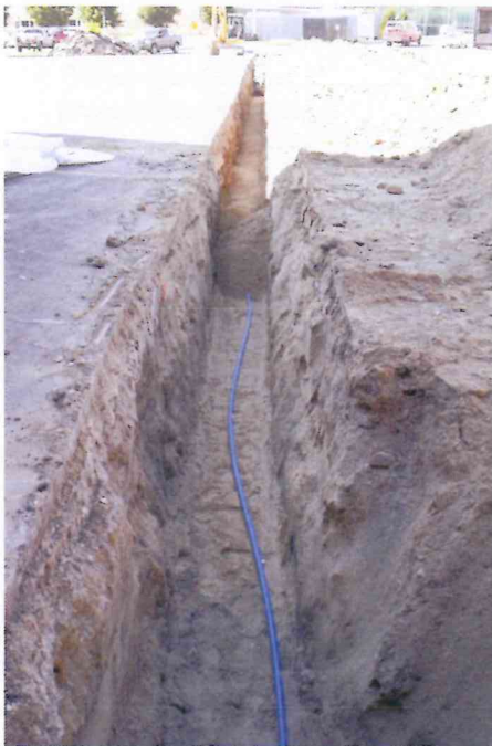
New Water Line to MHS
