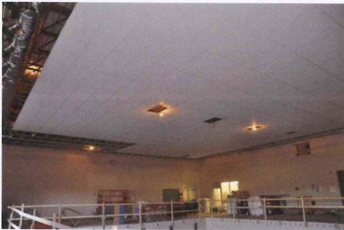
MHS – New ductwork and ceiling installed in pool
