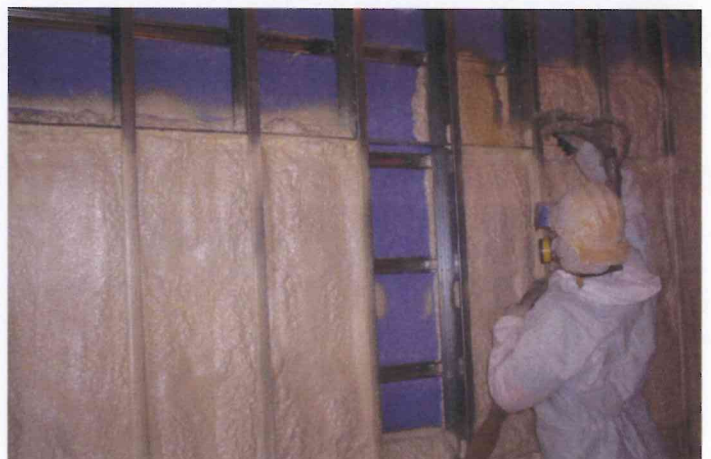
MHS – Classroom Addition Foam Insulation being applied
