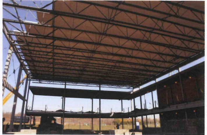
MHS – Gymnasium Addition roof panels being installed
