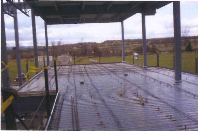
MHS – Gymnasium Addition mezzanine being prepped for concrete pour
