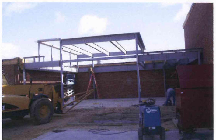
ES – Music Room steel being erected
