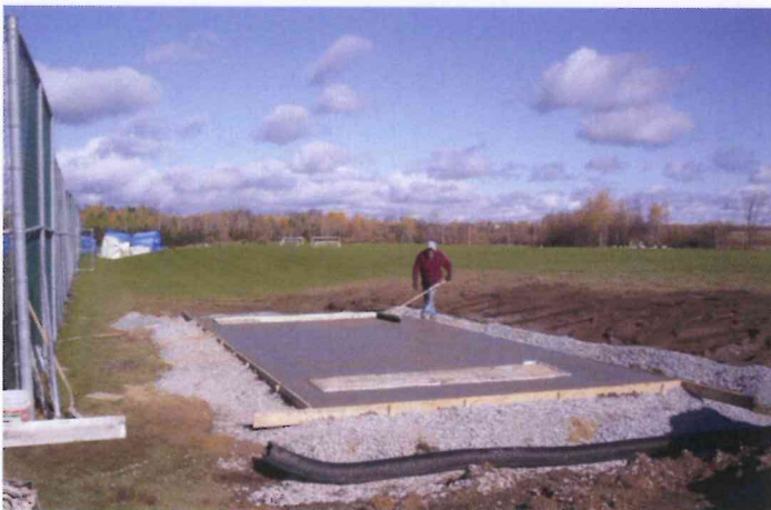
ES – New Fuel Oil Tank Pad being finished
