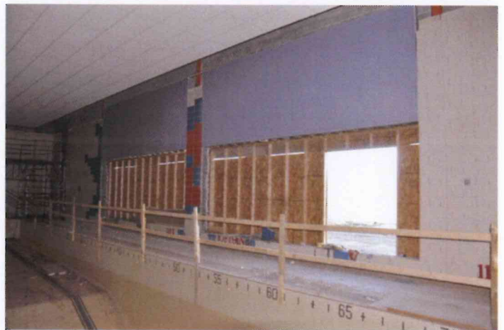
MHS – New window openings created in North wall of pool
