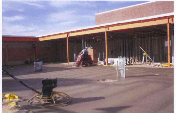
MHS – Finishing floor for Administrative Entrance & Offices
