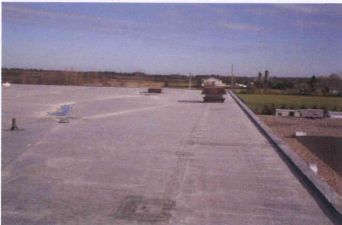
MHS – New Pool Roof
