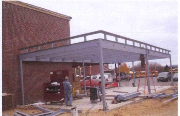
ES – District Office steel being erected
