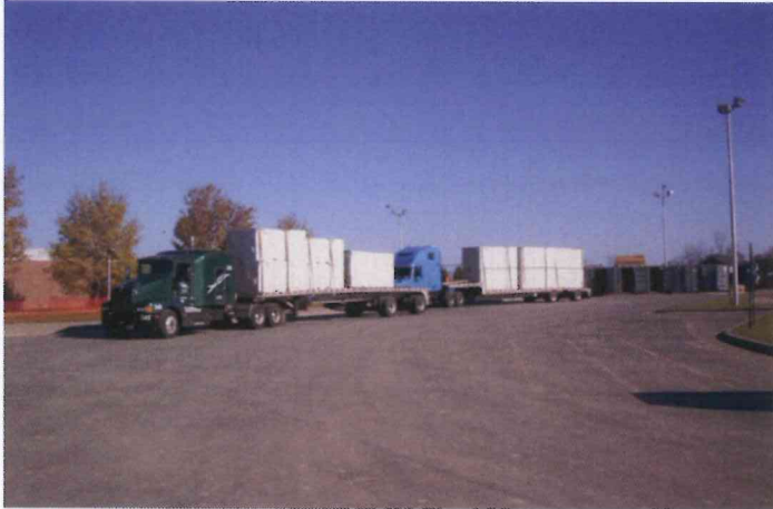
MHS – Roof top mechanical units arrive on site
