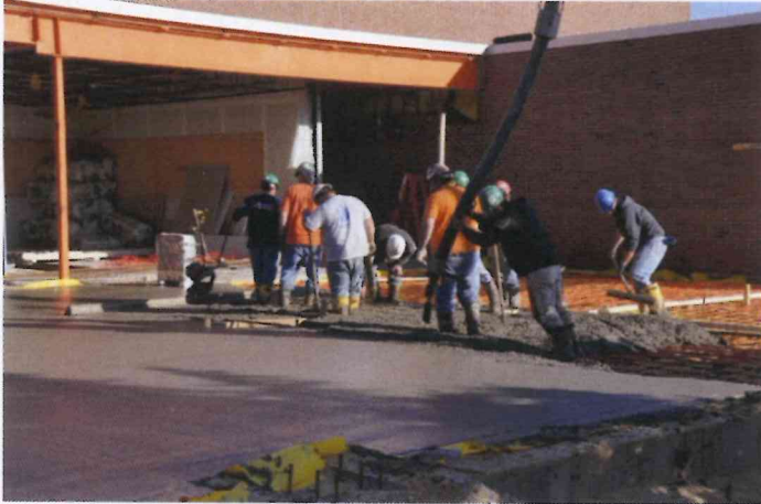
MHS – Pouring concrete floor for Administrative Entrance & Offices
