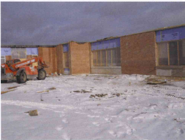
MHS – Classroom Addition exterior brick veneer
