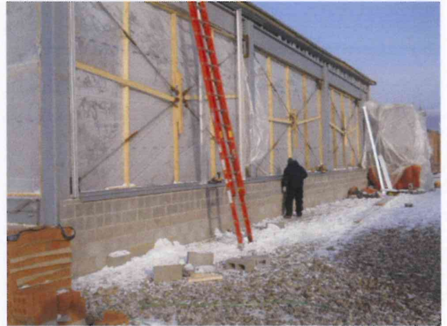
MHS – Gymnasium Addition south side window frames being installed
