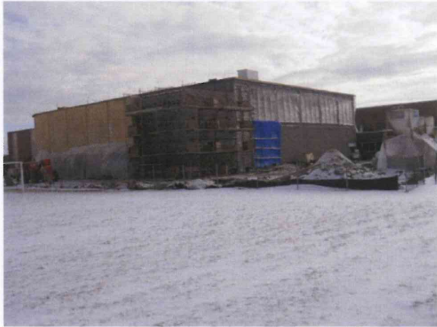
MHS – Gymnasium Addition enclosed for winter
