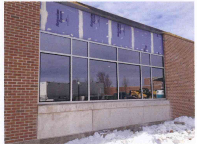
MHS – Classroom Addition first window installed
