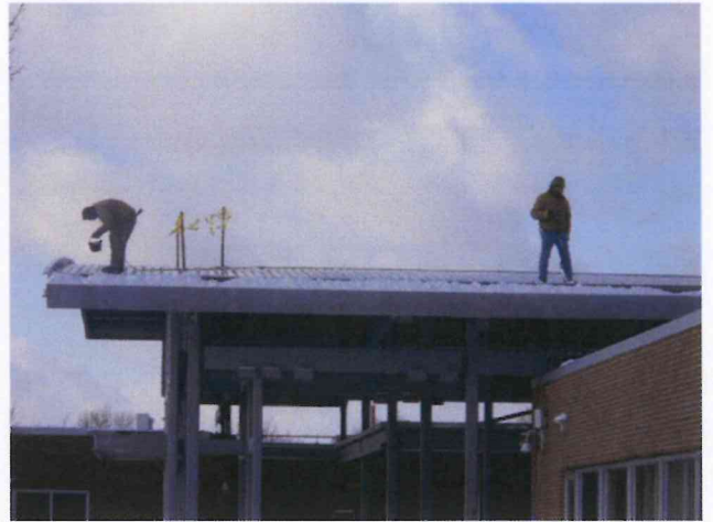
MHS – Main Entrance roof deck being installed
