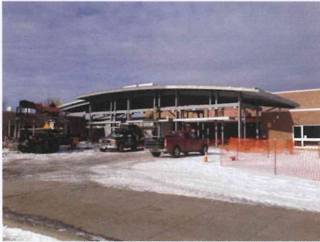
MHS – Main Entrance
