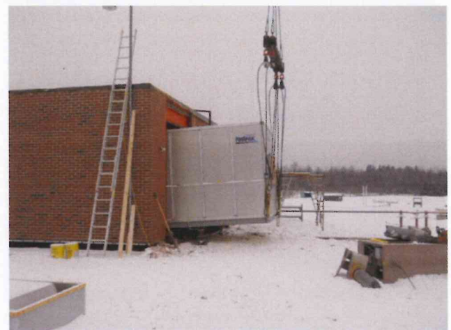
MHS – Pool Pak (HVAC) being installed through side of building
