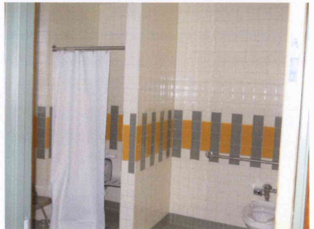
ES – Nurse's Toilet Room
